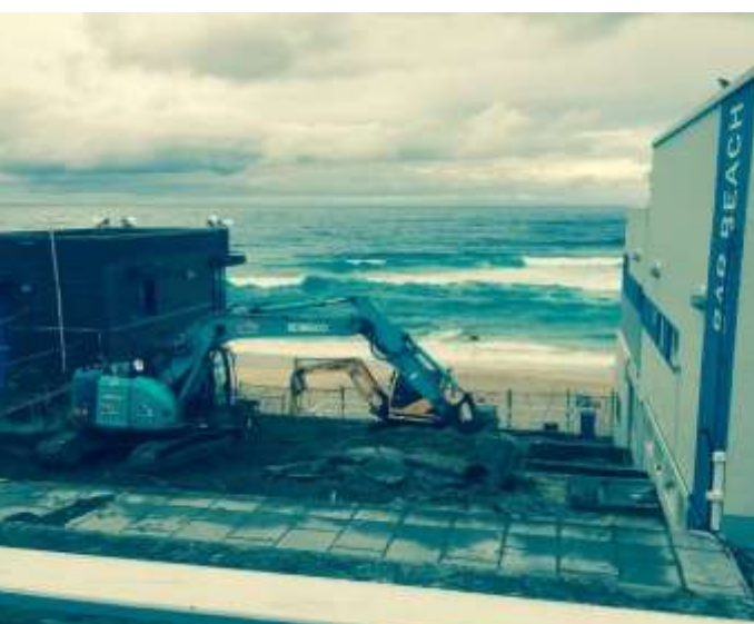
Excavation begins for the Surf Club extension – August 2016
