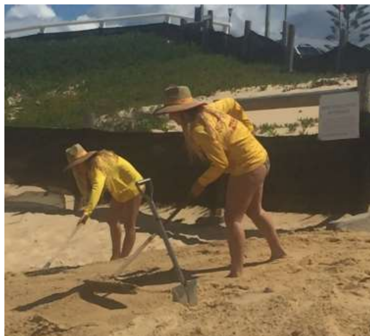
Patrol members fixing the ramp at the south end of the clubhouse
